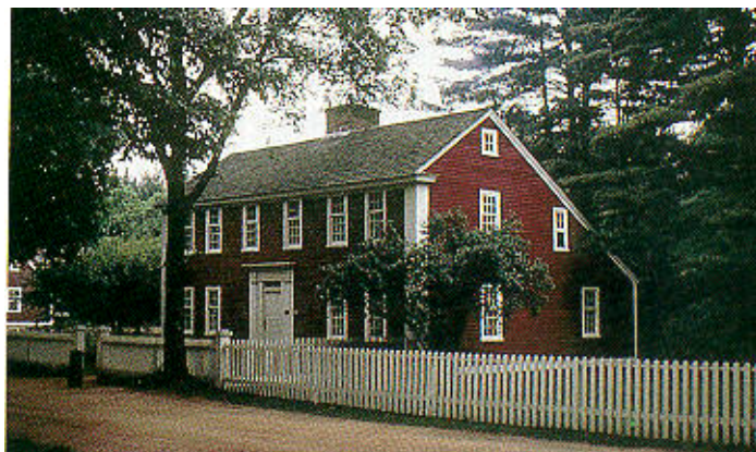
Saltbox House, New England, USA
